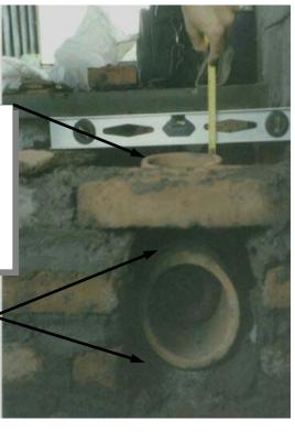
Once the elbow is positioned — 2" above the floor of the stove body, 1/2" below the exterior walls, and 3" from the front wall (see photo right) — join the 2 pieces of the elbow together with the same clay/sand mix that was used for mortar.
